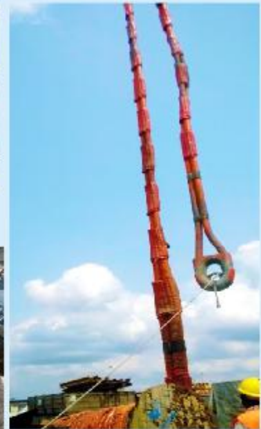
Mooring Grommet pre-installation Line-up
