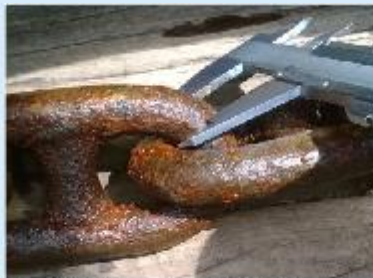
Hang-Off; Pick-up Chain Integrity Inspect on
