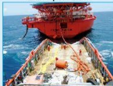
Installation of Mooring Hawser to FPSO Front PUFFIN
