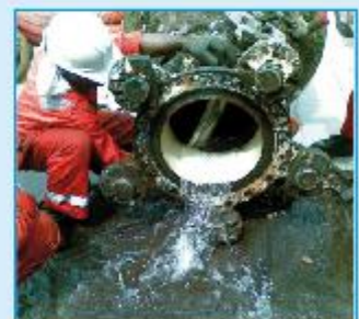
Floating Hose Back Flush Completed
