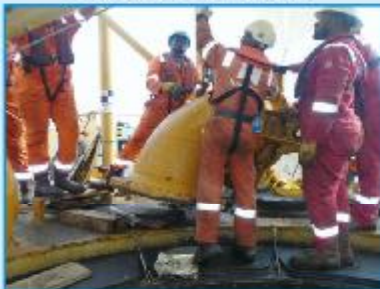
Bonga SBM Central Pipe Swivel Replacement
