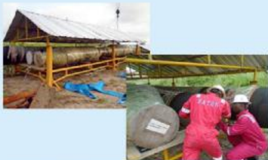
Hose Rack Storage Installation And Hose Alinging
