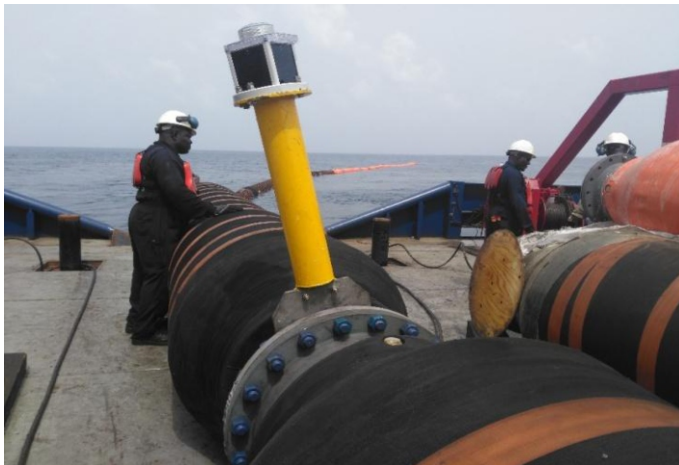
Chevron Project Jan 2018, Winker light installation on FHS.
