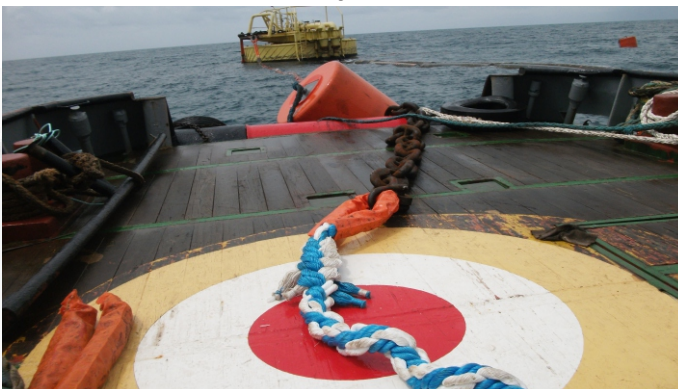
SPM Mooring rope inspection and maintenance
