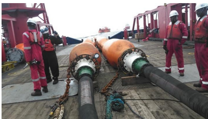
Chevron Project Jan 2018, Back flushing connection line up completed
