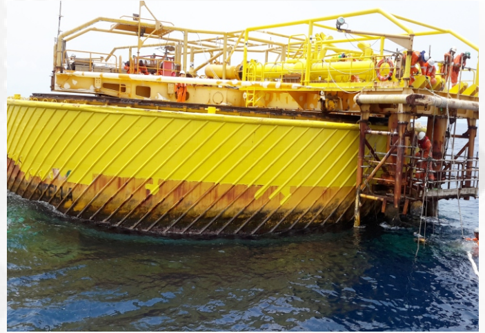
Bonga SBM Export Floating Hose Installation Leak Test
