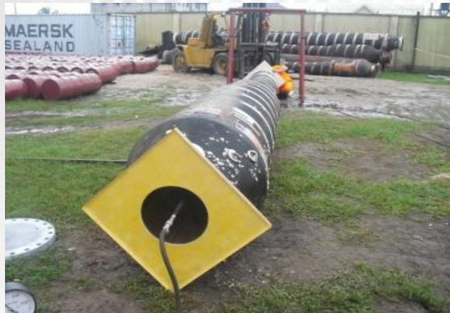
Export Hose Integrity Vacuum Test
